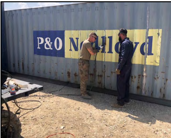
SGT Sarenana helps a Special Forces ODA Team create a close quarters combat training facility out of shipping containers using a plasma cutter.
